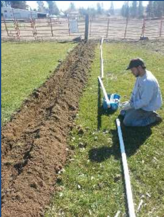
New Pipe Installation at Rodeo Grounds
