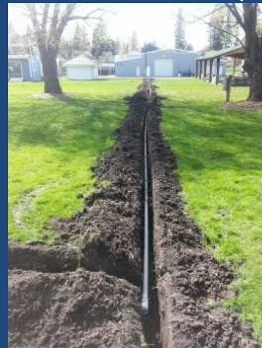
New Pipe Installation at City Park
