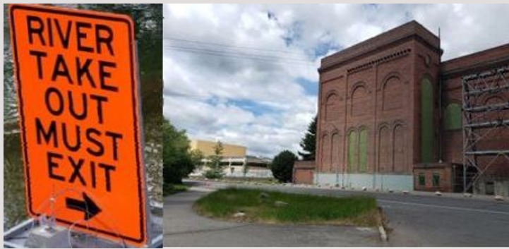
Take out river right at this building
