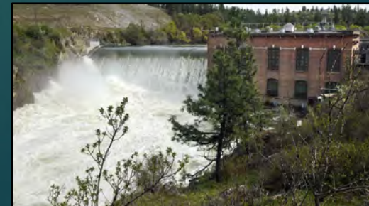
Nine Mile Dam, Avista Corp
