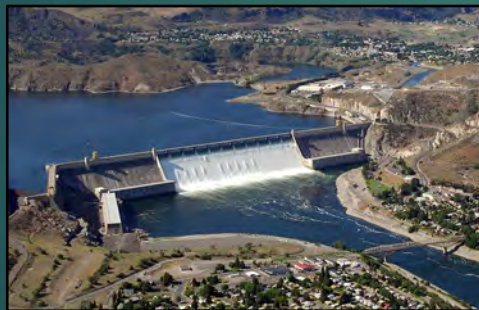
Grand Coulee Dam, BOR
