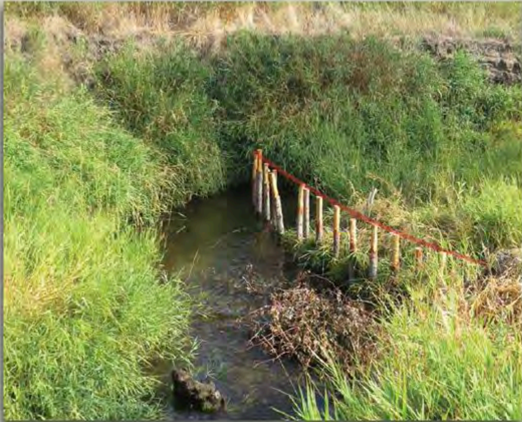
Before: Beaver Dam Analogue (BDA) #17 on September 7, 2016, right before it was woven. Note the red line along the post tops.
