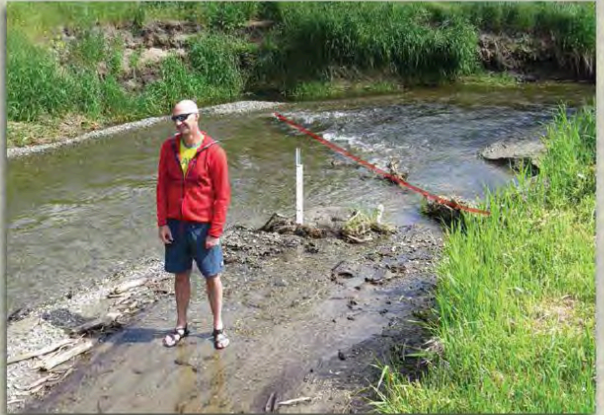
After: On June 22, 2017, Robes Parrish stands on top of 4.5 feet of aggraded sediment, in front of BDA17. Note the red line, at the new streamed elevation!
